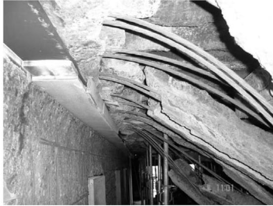
**Figure 1.2 – damage to the hollow core slabs in Rotterdam following a fire in a car park [20]**
