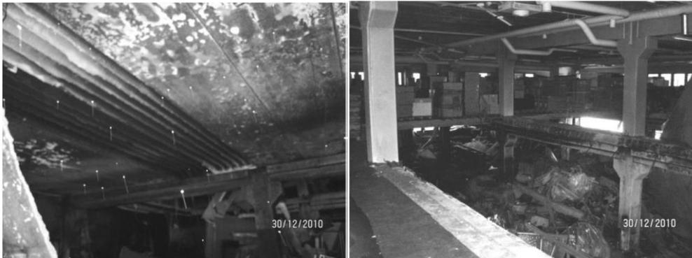
**Figure 1.3 – damage to the hollow core slabs in Vantaa, Finland; left shows delamination of the lower flange, right shows the void left following collapse of one of the floors [23]**
