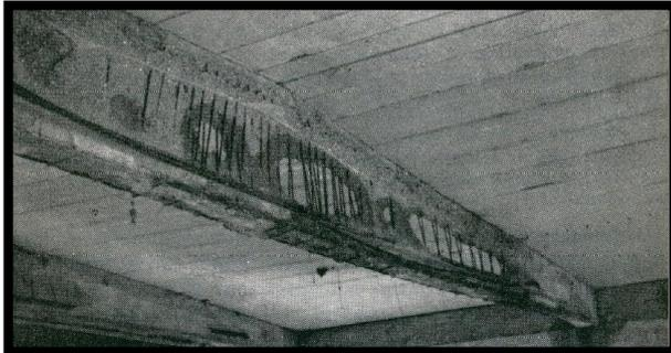
Figure 2.4 Spalling of pre-stressed beams due to fast cooling by adding water described by the Swedish Tariff Association (1959).
