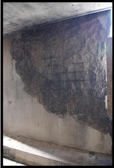
Figure 2.24 Fire spalling of the external wall of a garage. The heat source was three burning vehicles. Note the absence of spalling on the roof slab. The reason for the difference could be caused by (i) differences in concrete quality and/or (ii) difference in load situation where the wall element is loaded in compression. Photo Robert Jansson.
