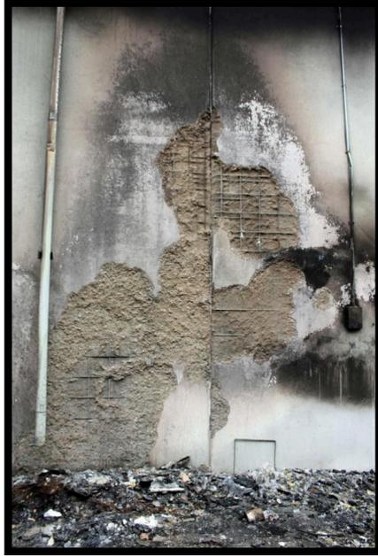
Figure 2.22 Fire spalling on an external concrete wall. The heat source was a burning tractor. Photo Robert Jansson.
