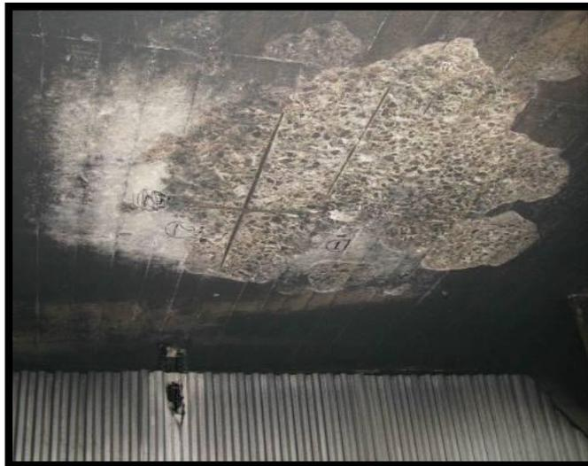
Figure 2.23 Fire spalling in the roof in a garage. The heat source was a burning car. Photo Robert Jansson.
