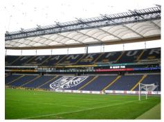
translucency and their potential for architectonic expression. However, a common limitation on all textile materials is their fire behavior, which emphasizes the importance of correct fire safety assessments when using such materials in building structures.
