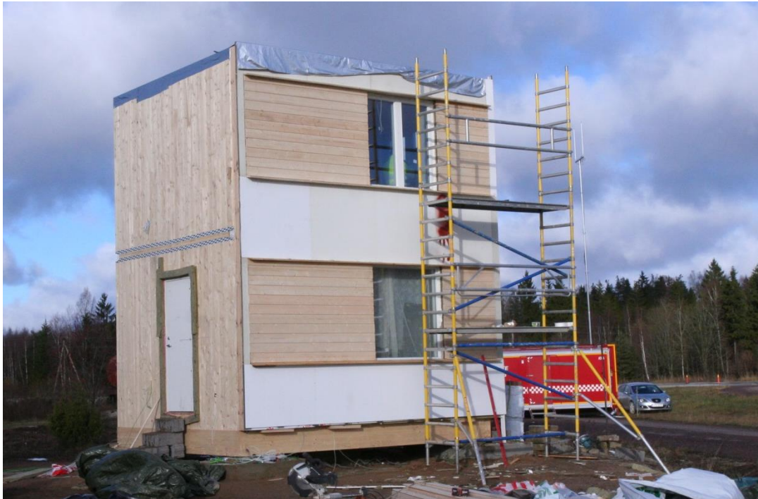
Figure 35: Façade of the building with timber panels and non-combustible cement board strips.
