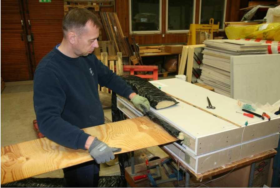
Figure 24: Sliding fire stop into the cavity for a U-shaped placement
