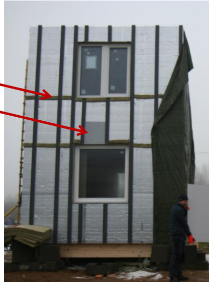
Figure 34: Fire stops installed during the construction phase
