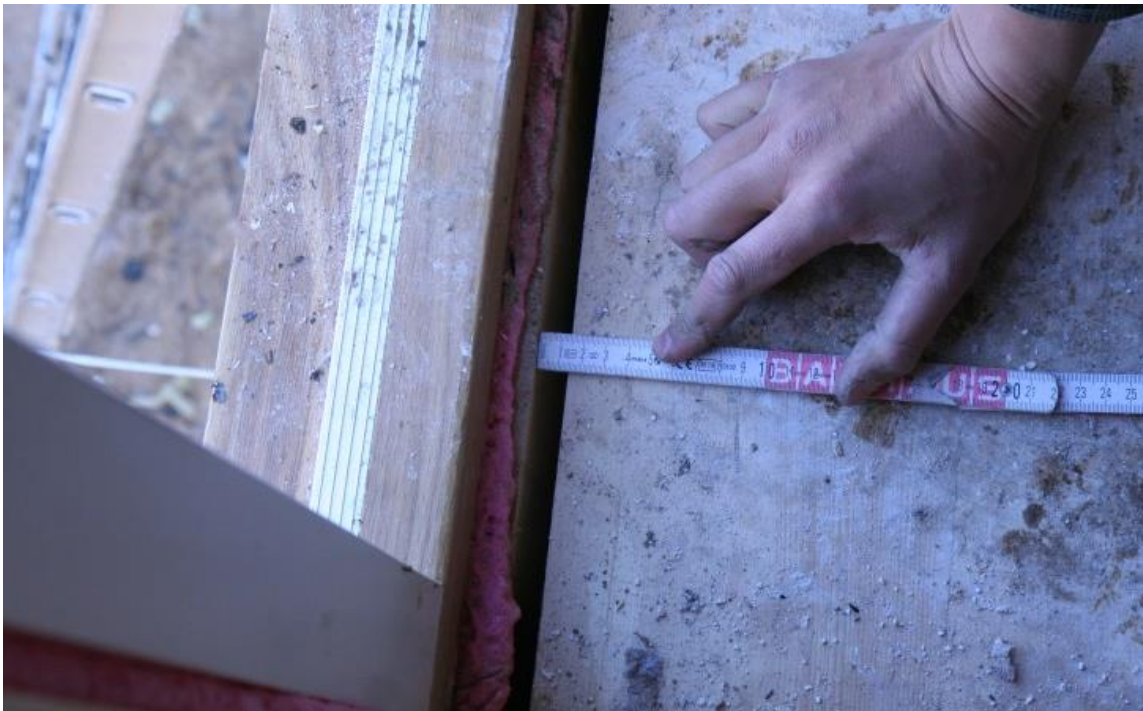
Figure 31: maximum gap measured (14mm) in between wall and floor slab
