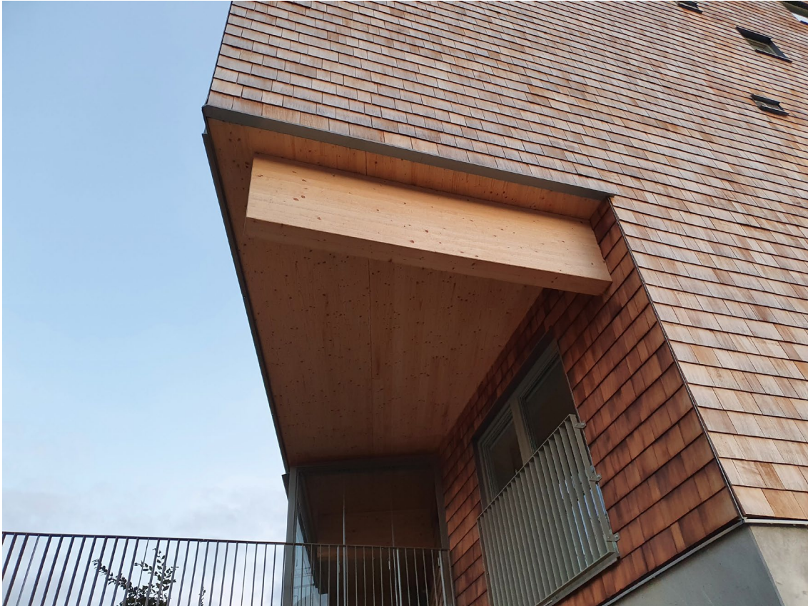
Figure 4: Picture of a floor slab extension with exposed timber above a balcony in a residential building with wooden façade. (Photo Carl Pettersson)
