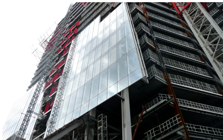
Figure 18 Curtain walling system under construction. (Picture courtesy Steelconstruction)
