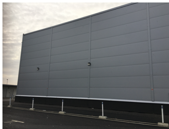
Figure 15 Example of a sandwich panel system (picture Patrick van Hees)
