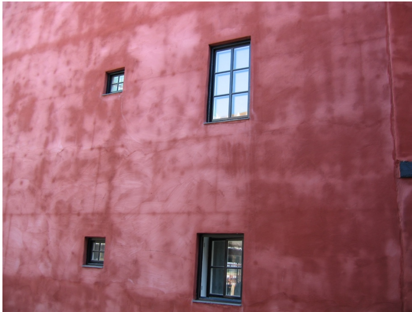
Figure 14 Example of an ETICS system (thin render on EPS) (picture Miklos Molnar)
