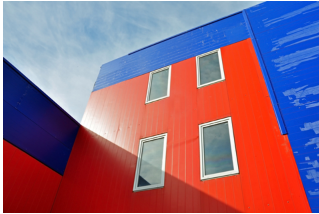
Figure 16 Example of a building with sandwich panels (picture ID 76945687 © Viktoryia Strukouskaya Dreamstime.com)
