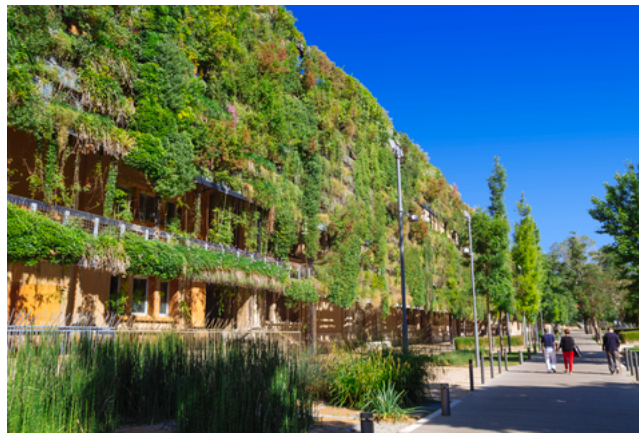
Figure 24 Example of a green façade system by adding plants on the outside of the façade (picture courtesy ID 64493637 © Jordi Clave Garsot | Dreamstime.com )
