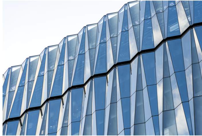
Figure 17 Example of a curtain walling system with glass panel (Image ID: 158518730 Copyright Askar Karimullin Dreamstime.com)
