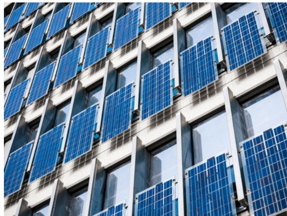
Figure 22 Example of solar system integrated in the façade (picture courtesy ID 152117419 © Vtt Studio | Dreamstime.com)
