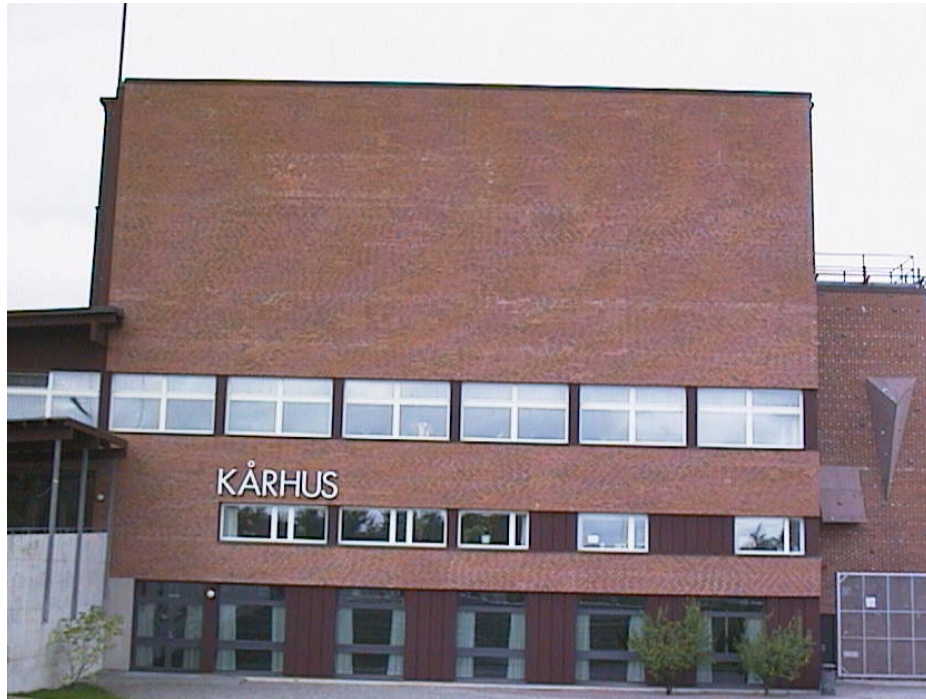
Figure 10 Example of a brick veneer building – LTH administration building (picture Lund University)
