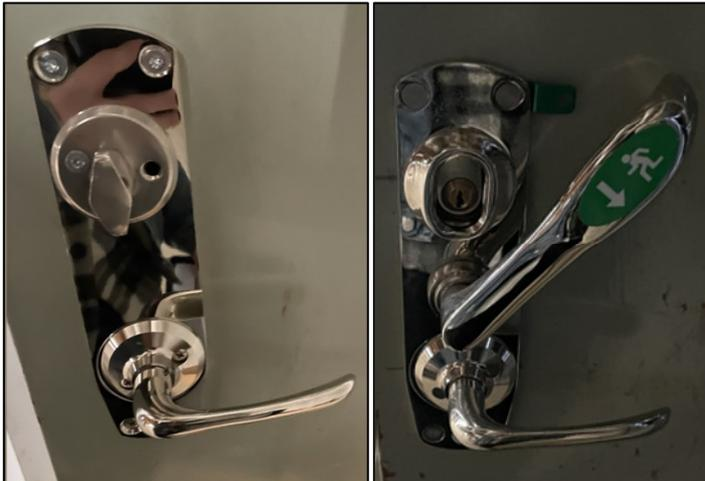
Figure 3. Design of door fittings. Inward opening side to the left, and outward opening side to the right.
