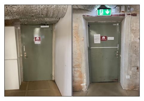
Figure 2. Design of the door. Inward opening side to the left, and outward opening side to the right.
