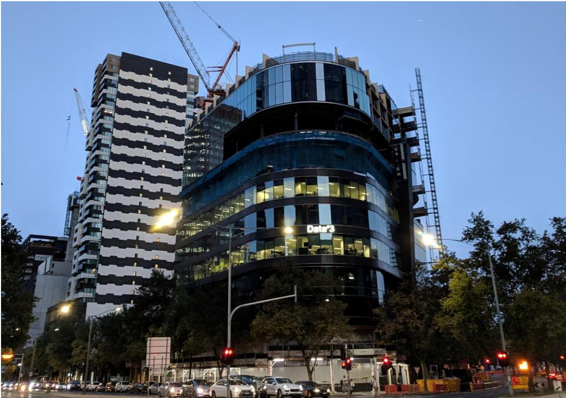
*Figure 10: Example of mass timber construction being used to construct a ten-storey hotel on top of an existing building. (Photo Carl Pettersson)*
