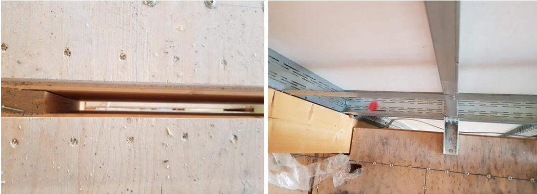
Figure 9: Example of gaps in floor slab (left) and curtain wall system (right) in a timber building during construction. (Photo Carl Pettersson)
