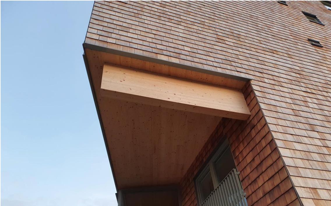
*Figure 5: Picture of a floor slab extension with exposed timber above a balcony in a residential building with a wooden façade. (Photo Carl Pettersson)*
