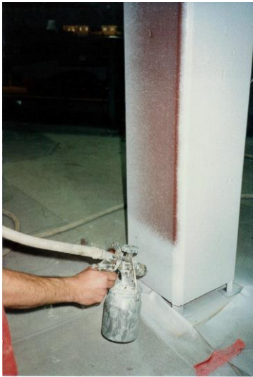
Figure 1 Application of a intumescent system on a steel column.
