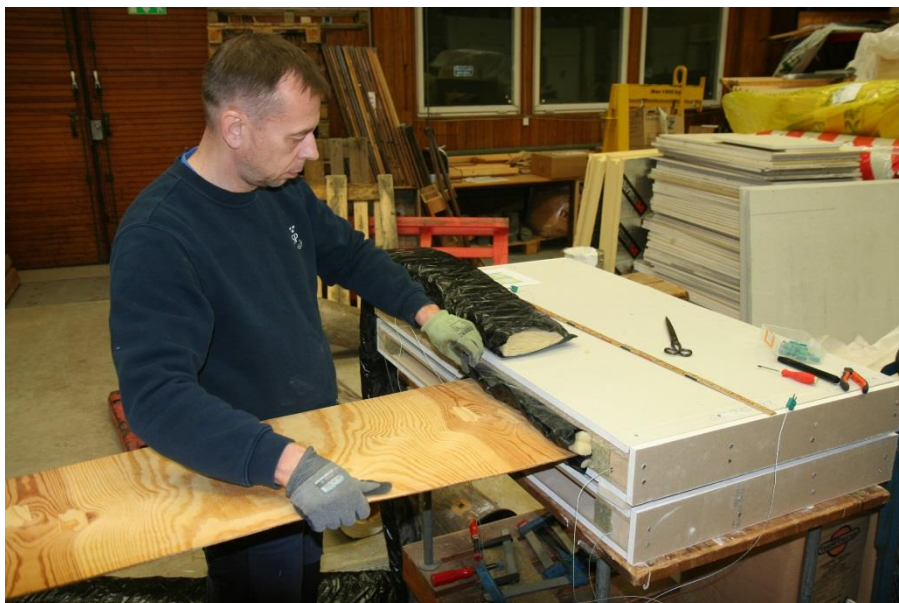
Figure 23 - Sliding cavity barrier into the cavity for a U-shaped placement
