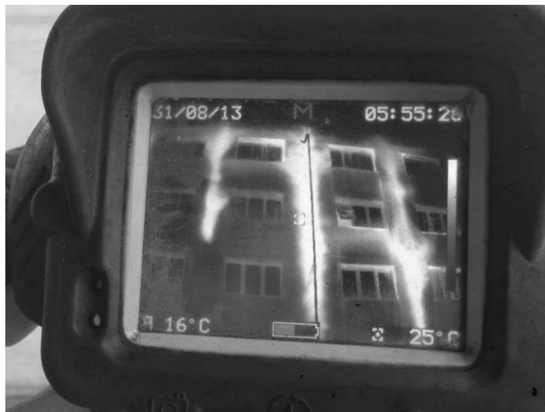
Figure 5 -Infrared camera picture indicating a downwards fire spread through cavities 2
